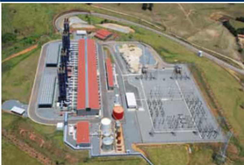
TEVISA – VIANA THERMOELETRIC POWER PLANT
