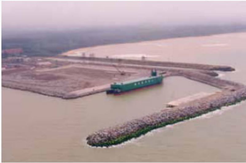
ARCELOR MITTAL TUBARÃO – OBT (OCEAN BARGE TERMINAL) – TURN KEY PROJECT
